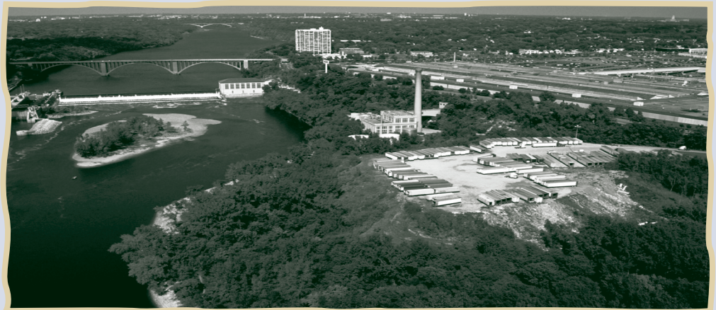
Roughly 4,000 housing units and a stream-like water corridor will be built along the bluff near the Ford dam in St. Paul, but open space and pollution concerns linger. The toxic dump known as 'Area C' is featured in the foreground above. (Photo courtesy of the Regents of the University of MN)
