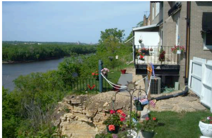
This development in Lilydale was built much too close to the bluff (prior to the establishment of MRCCA) creating serious and costly bluff erosion problems, as well as scenic impacts.
