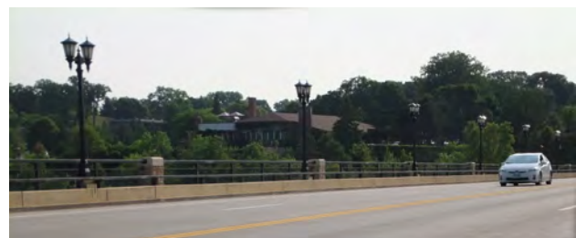
Figure 4. View of the Town and Country Club on the east bank from the Lake Street/Marshall Avenue Bridge
