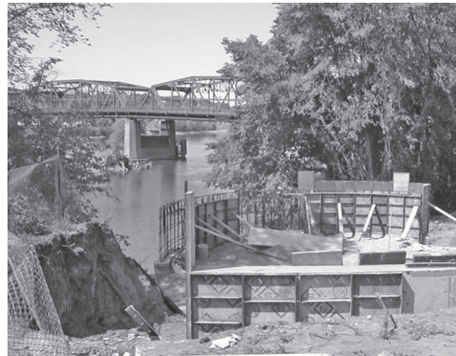
Construction of a Mississippi River overlook was underway this summer at the new Edgewater Park in northeast Minneapolis. In addition to great views, park visitors can enjoy trails, plantings, innovative stormwater treatment features and a restored shoreline.
