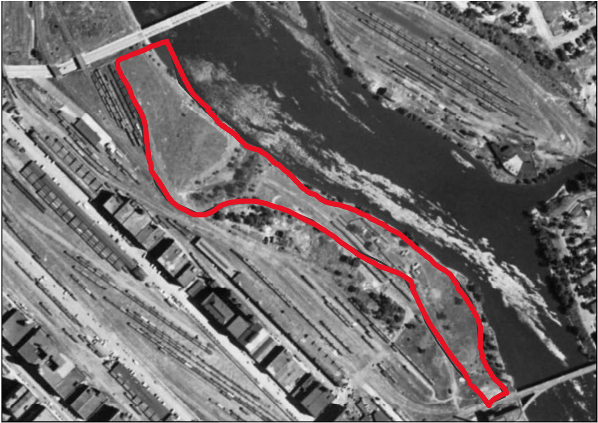
Figure 4: Historical Aerial Photography – 1940. James Rice Park Area Source: Hennepin County Aerial Imagery.
