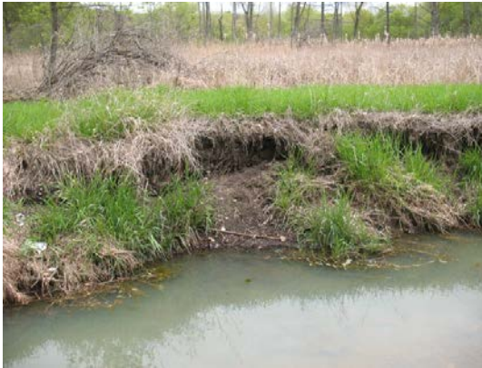
Photo 3. Severe bank erosion on stream that emanates from Beltway Pool in LHF-1.
