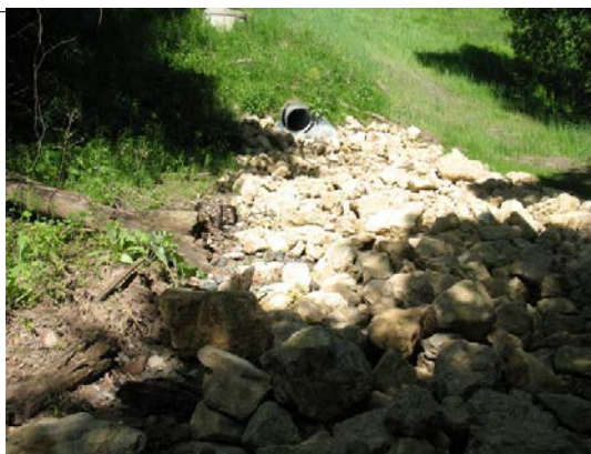
Photo 5. Inlet pipe with rip rap located at northwest end of LHF-2 unit. Slope in background is the berm from Highway 61.
