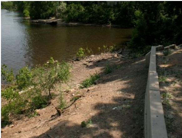
Photo 22. "North Corner" of Bassett Creek confluence with the Mississippi River. Note the extensive bare and loose soil near the wall. Also note the wide bare soil shores on each "corner" of the mouth of the creek, indicating that significant erosive forces must be at work here.
