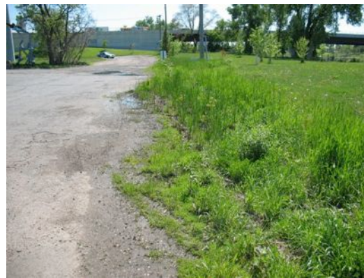
Photo 15. Boundary of parking lot and park; stormwater runoff pools here—note the darker gray water stains. Opportunity for infiltration.
