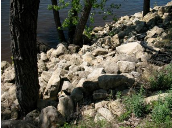
Photo 17. Heavily riprapped toe of riverbank. Little to no vegetation currently exists. Could try planting willow stakes into riprap.
