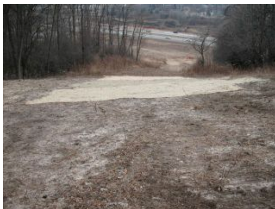
Photo 29. South end of pipeline right of way. Disturbance on slope and surface repair via erosion control blanketing.
