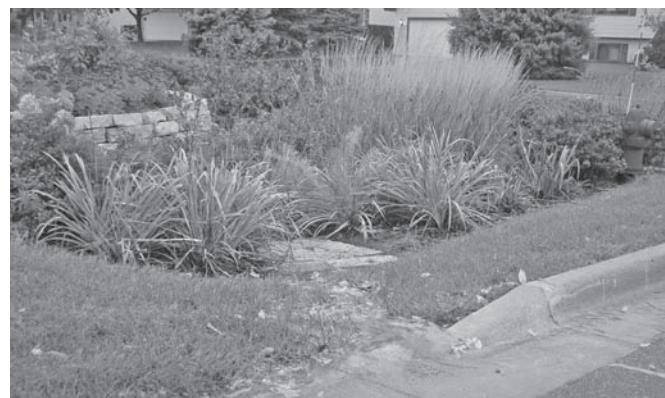
Rain gardens, like this one in Burnsville, are planted in a shallow depression with native vegetation to capture runoff and draw out pollutants. Photo: Barr Engineering
